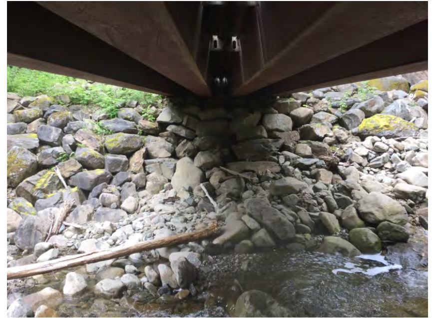
Right Bank Abutment when facing downstream
