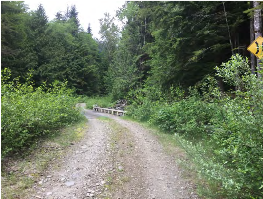
Approach from Left Bank when facing downstream
